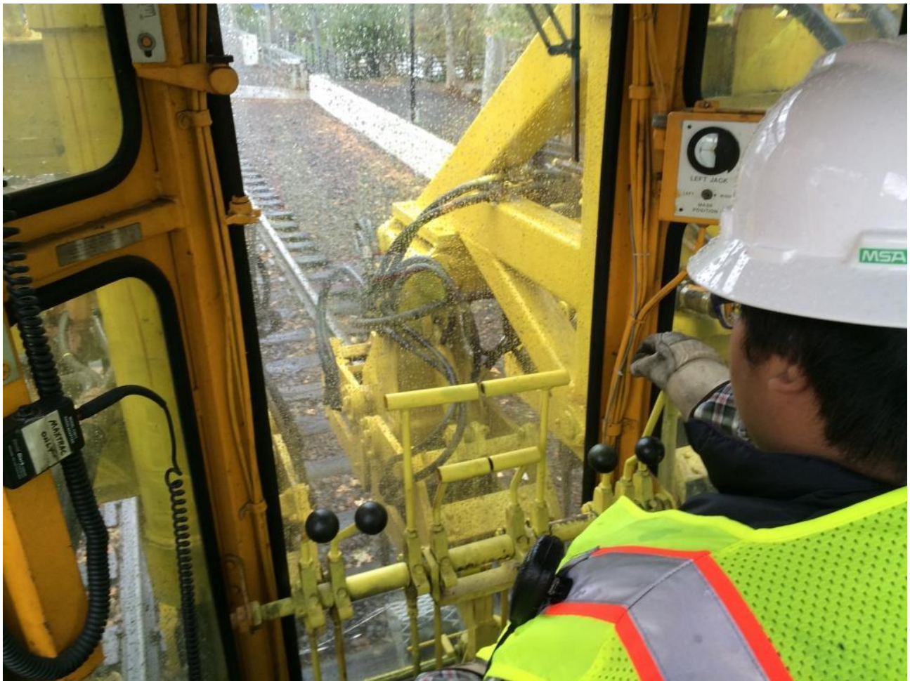
Anthony gets a lesson in tamper operations
