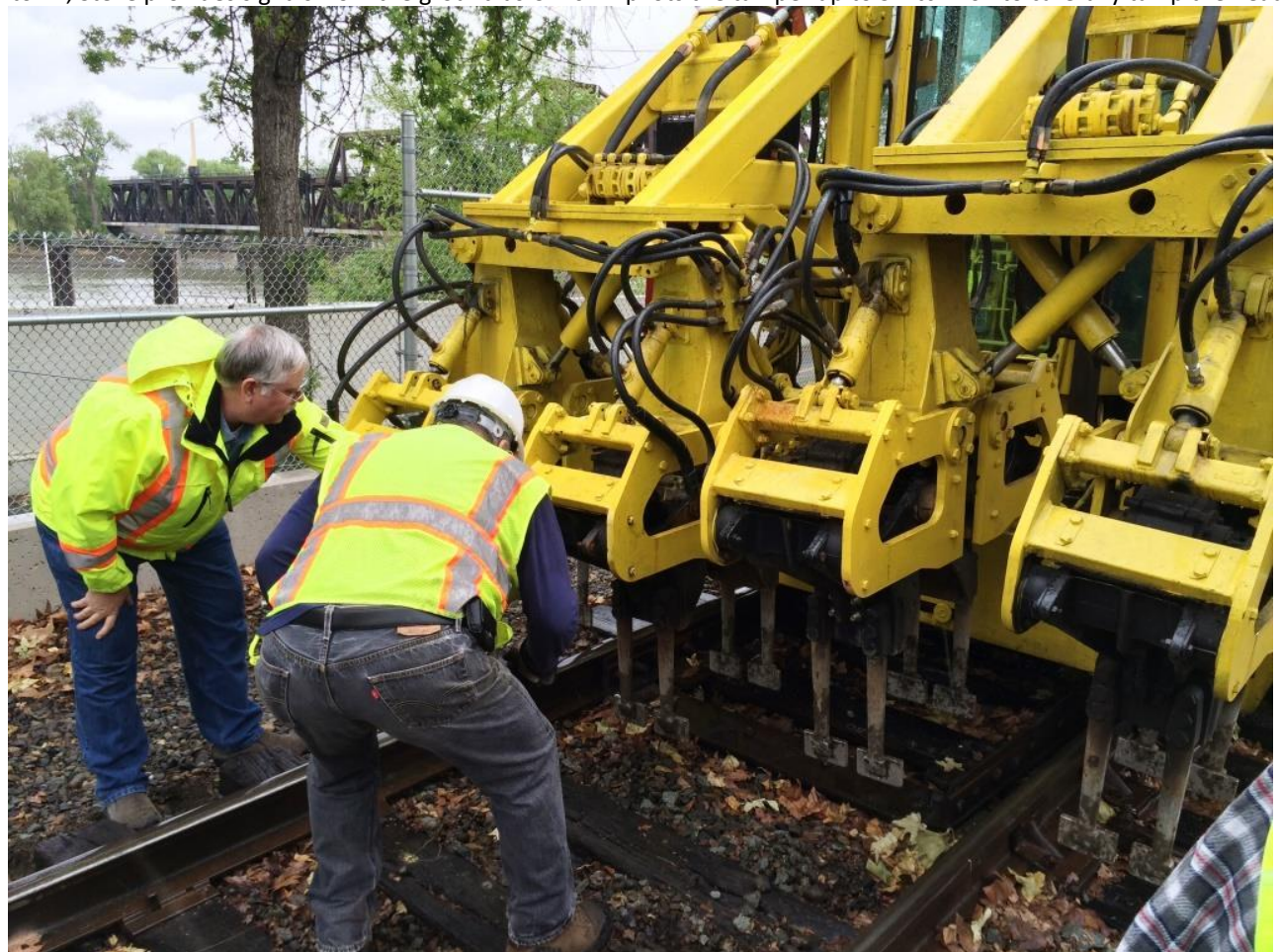
Chris C. and Steve closely monitor the tines as the descend around critical switch components
