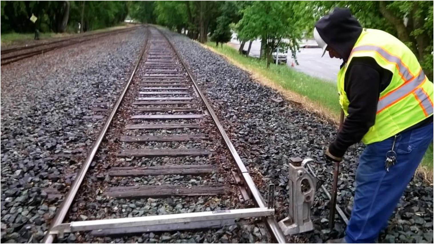
Harry sets a jack at a location where the west rail is low
