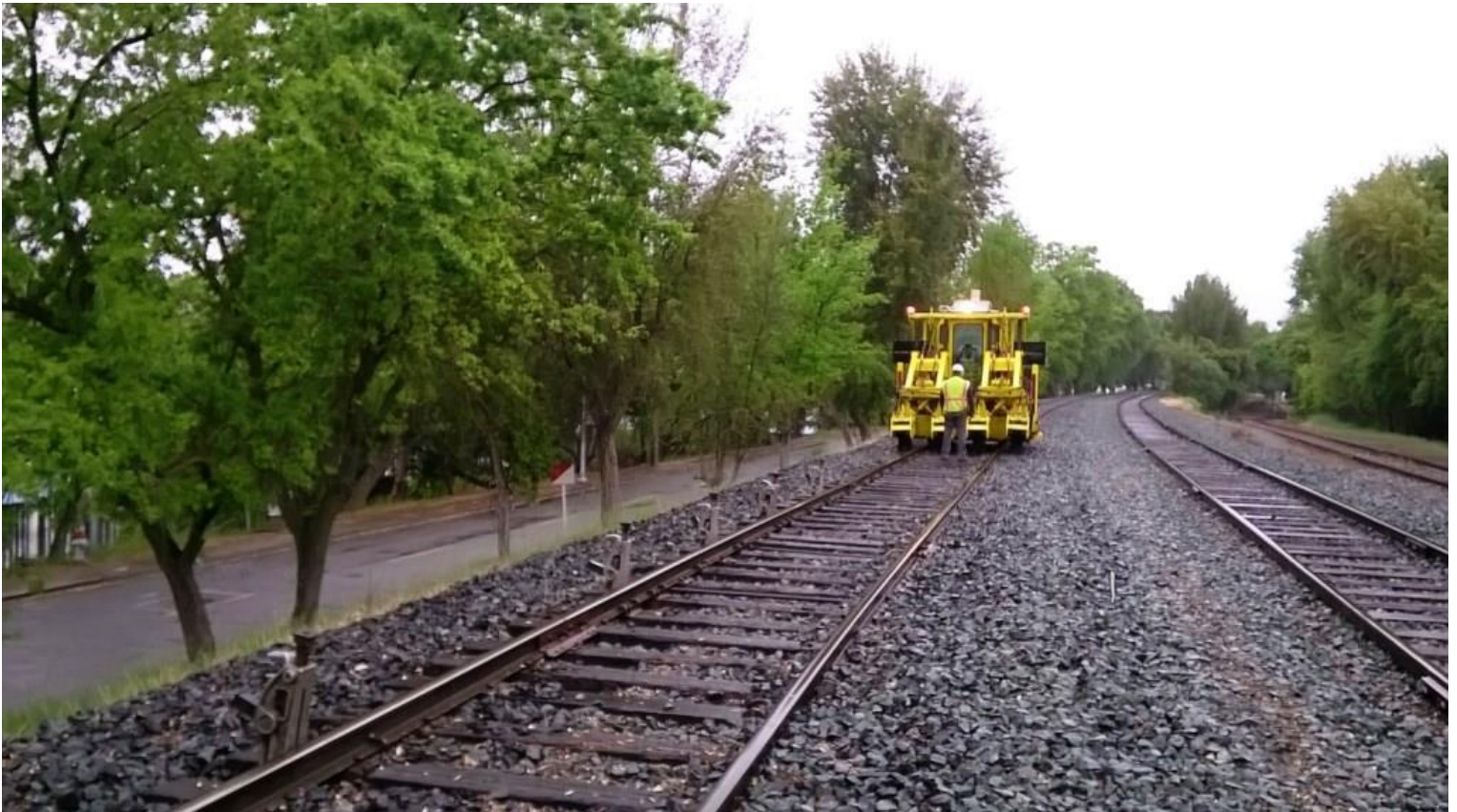
With all the jacks lined-up, the super-elevation was restored to the curve and Chris M. and Steve tamp the track to the new level
