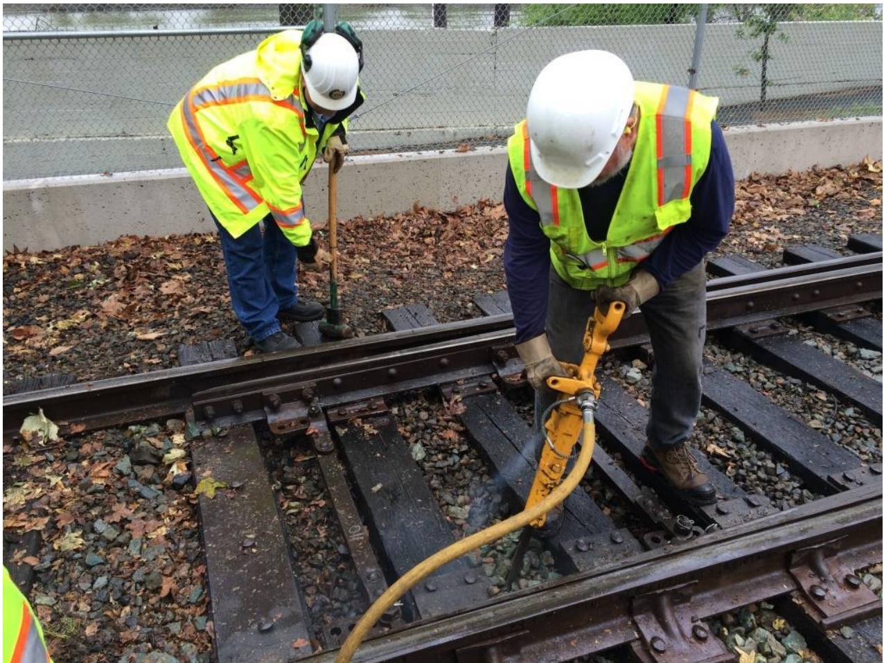
Steve hand-tamps switch-ties as Chris C. give the switch-plates a "ka-bang" with the ka-banger tool
