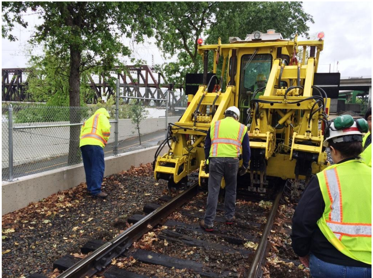
Chris C. and Steve keep a close eye on the switch-bits as Chris M. tamps-up the head-block
