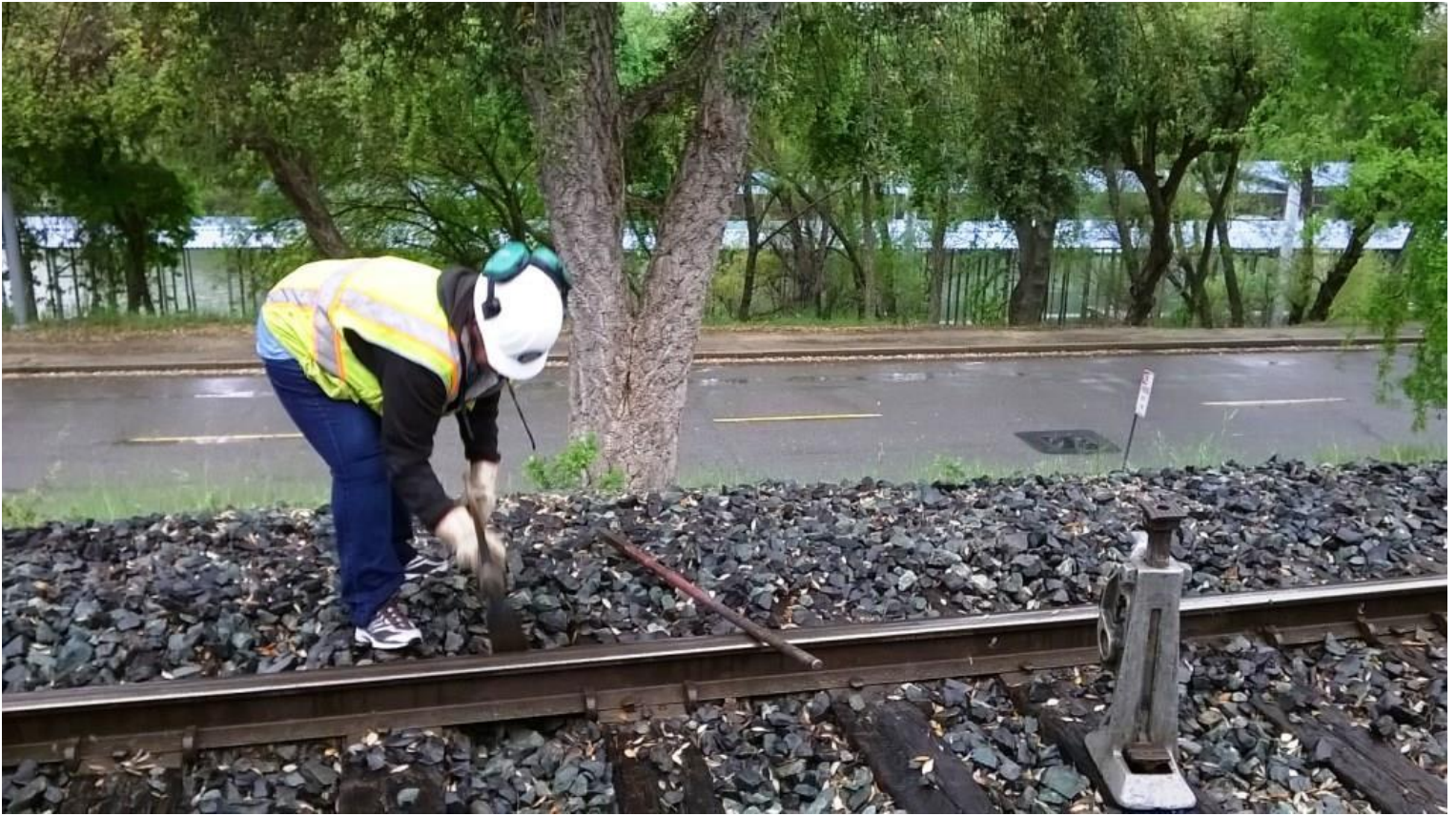
Pam uses a mattocks-tool to dig under the base of the rail in order to set a jack
