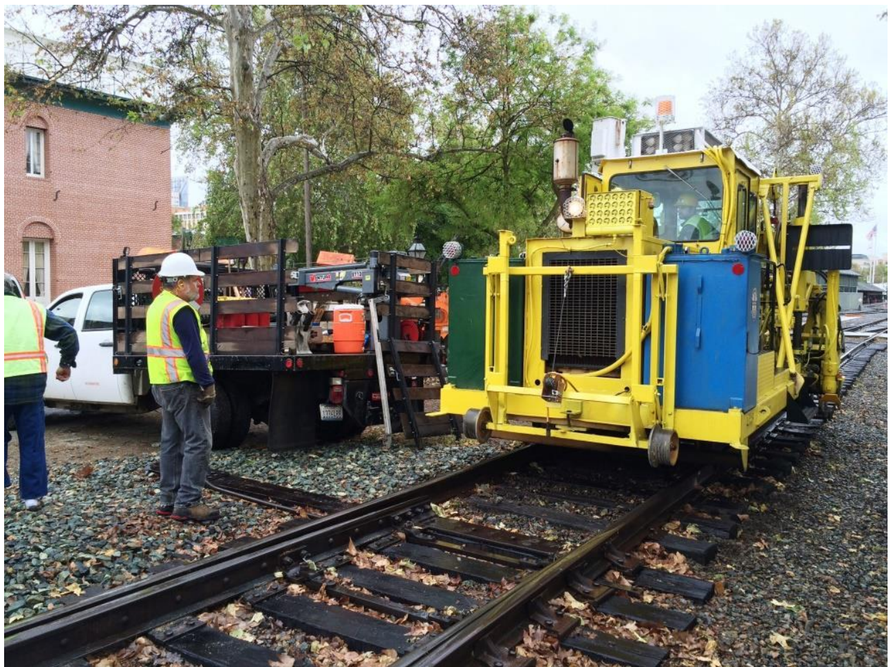
Back in town, Steve provides signals from the ground as Chris M. pilots the tamper up to Switch 101 to carefully tamp the head-block
