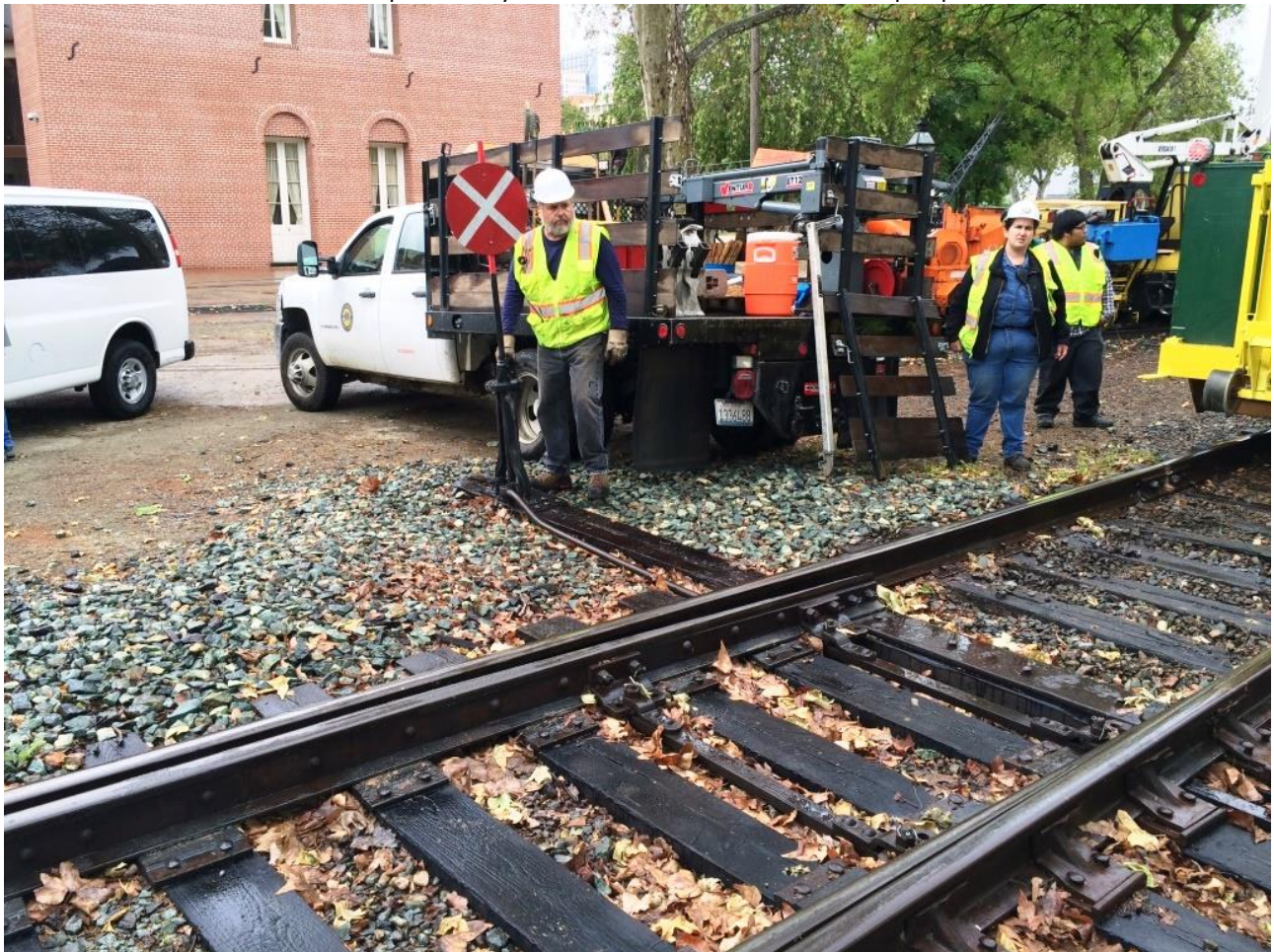
Steve throws the switch to see if tamping the head-block made any difference
