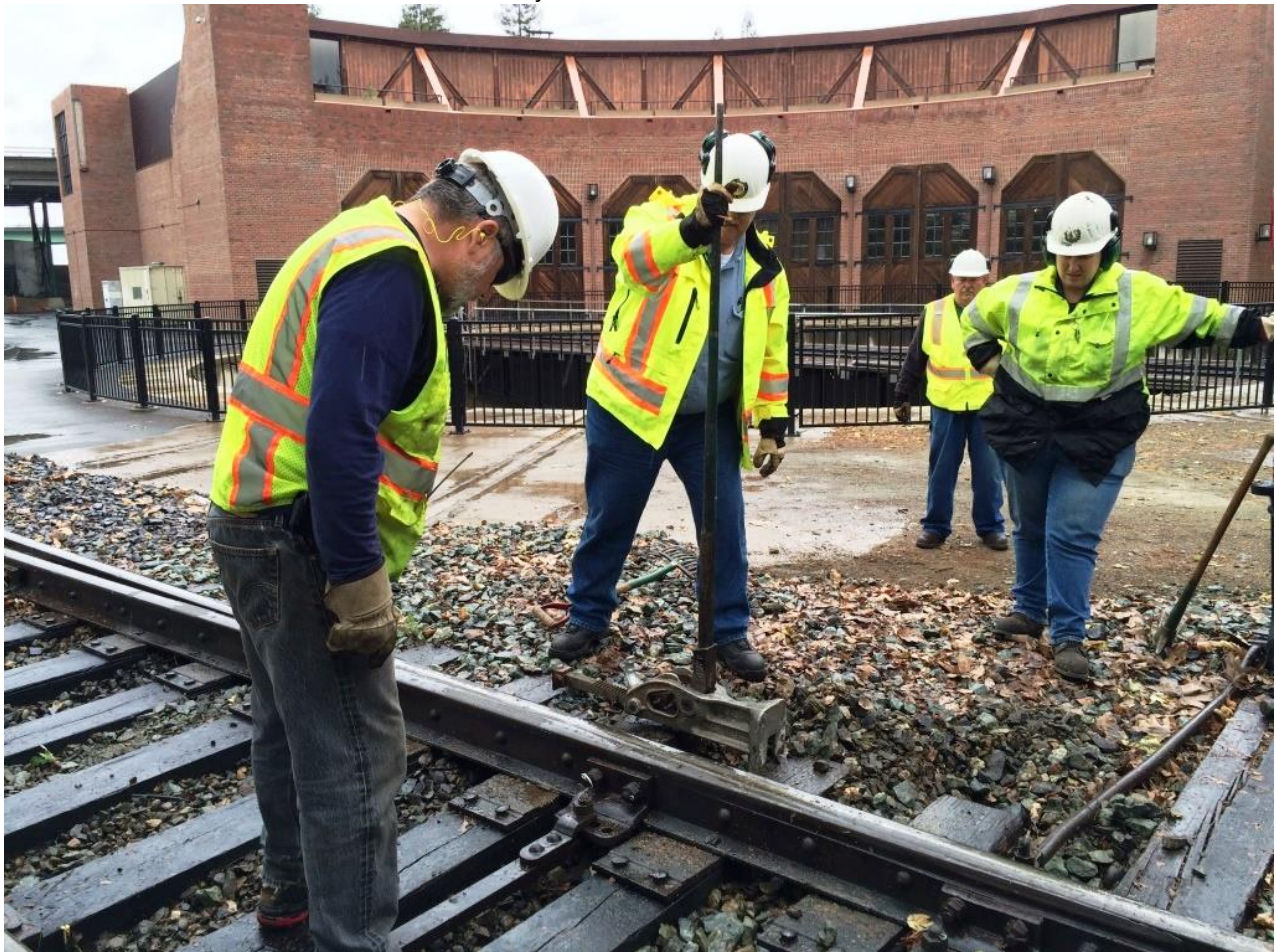
Now Chris C. tries to straighten catawampus ties with a track-jack
