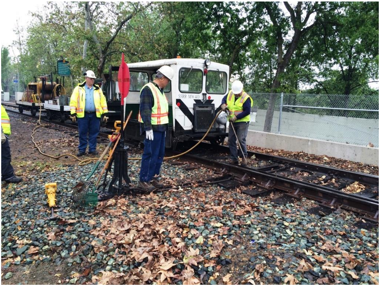
Steve uses the air-wand from the air-compressor to blow-out debris from switch-bits
